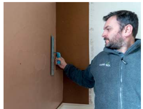
Plaster skim directly over the SprayCork
